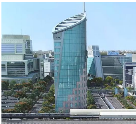
Figure: 1.1. DLF Gateway Tower, circular arc airfoil building, Gurugram, India
