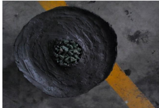
Figure 3. Ordinary floating Stone Column
