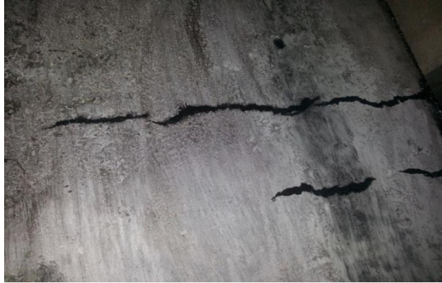
Fig.8 Crack sealed with resins and hardener
